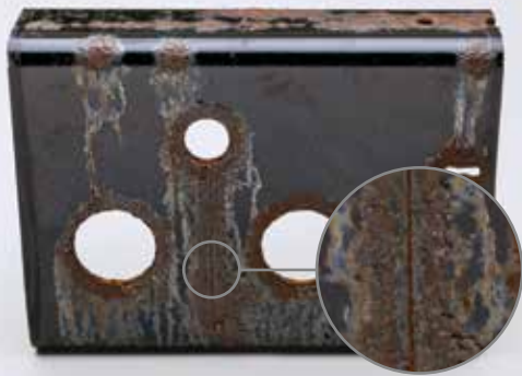
Significant rusting and blistering
